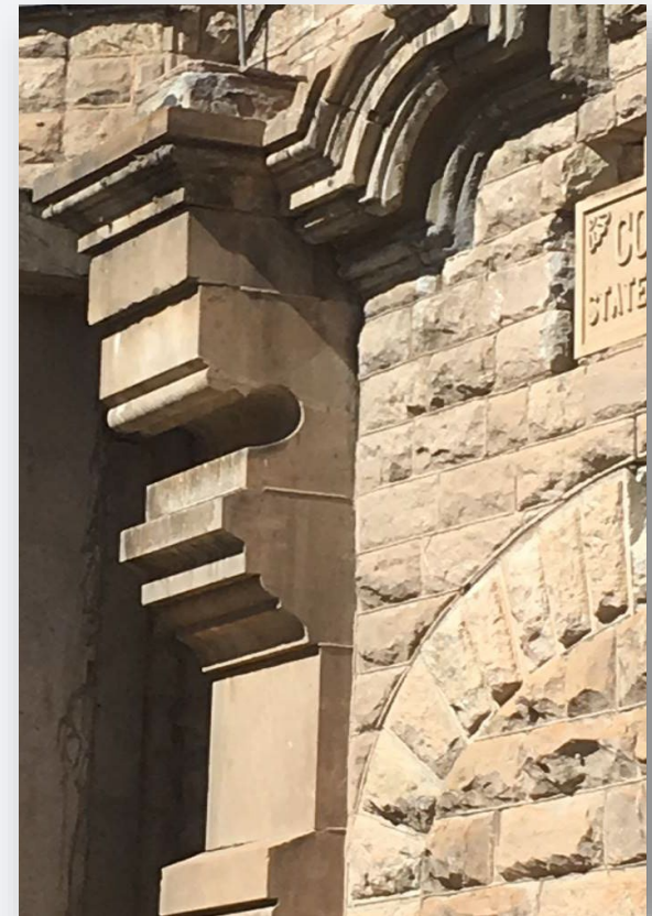
Colorado Territorial Correctional Facility Original Main Entry details
