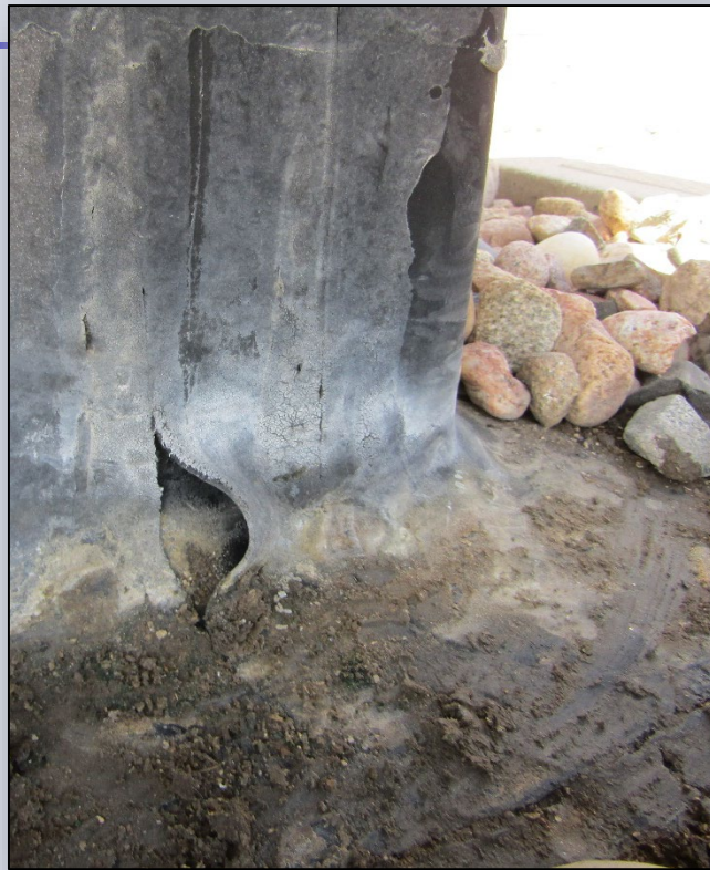
Denver Women's Correctional Facility Roof conditions
