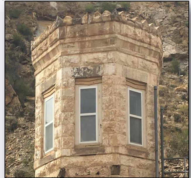
Colorado Territorial Correctional Facility Security Tower
