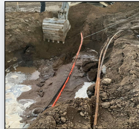
Buena Vista Correctional Facility Broken water line excavation
