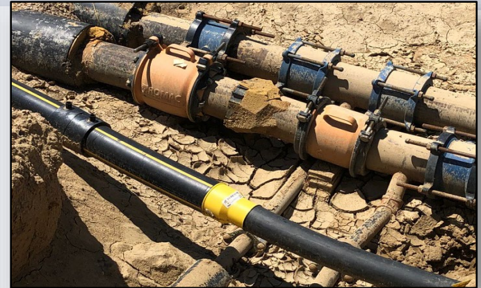
Arkansas Valley Correctional Facility Temporary water line patches
