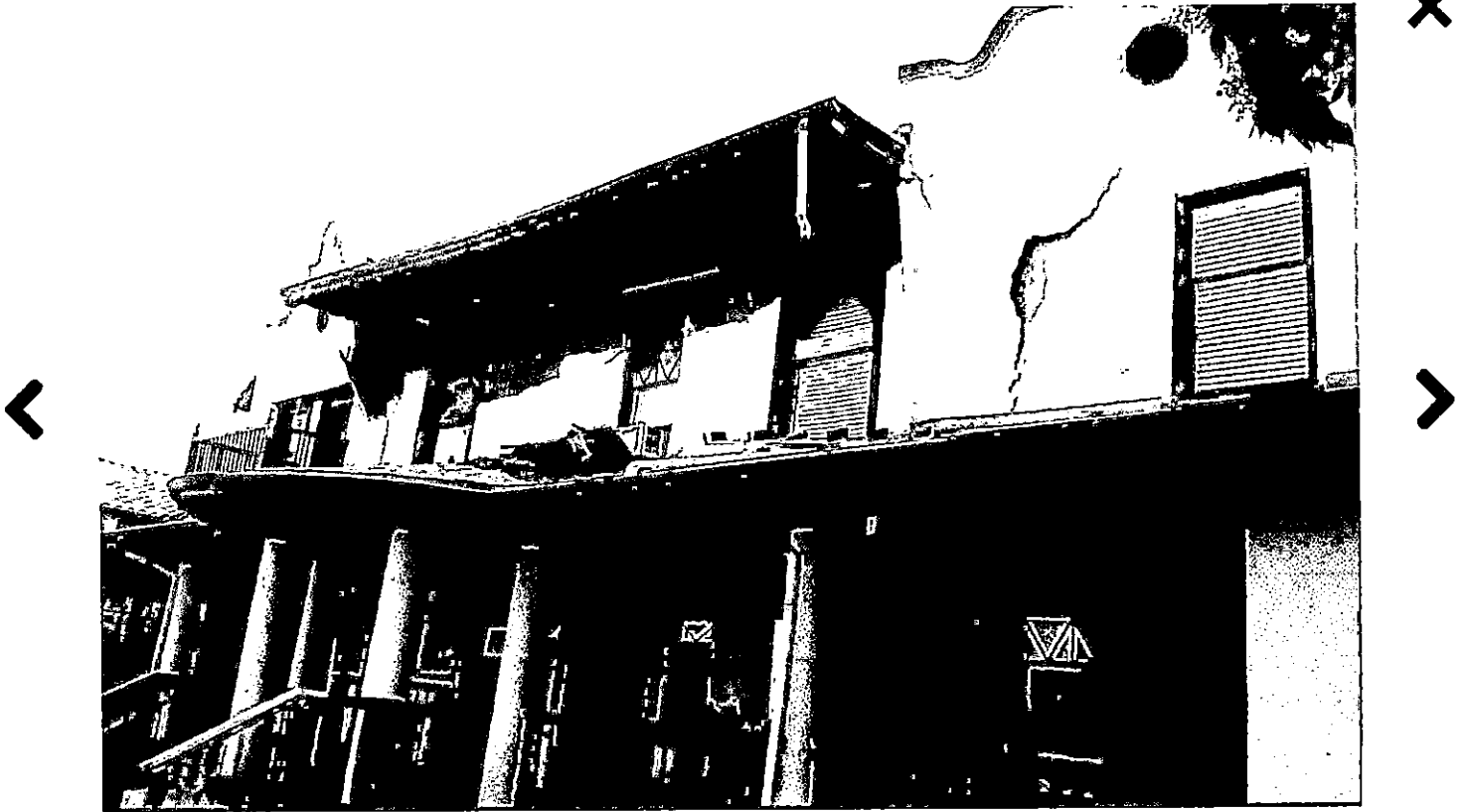
Partial building collapse 1646 Winona Court in Denver. Photo: Denver Fire Department
