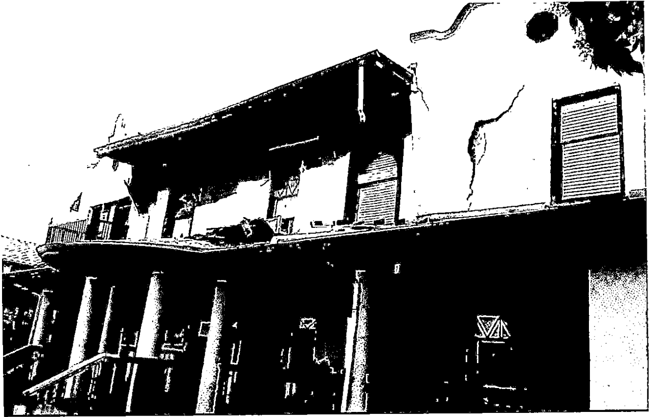
Partial building collapse 1646 Winona Court in Denver. Photo: Denver Fire Department
