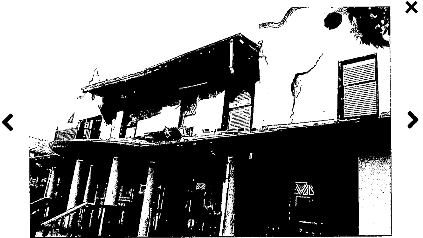
Partial building collapse 1646 Winona Court in Denver. Photo: Denver Fire Department
